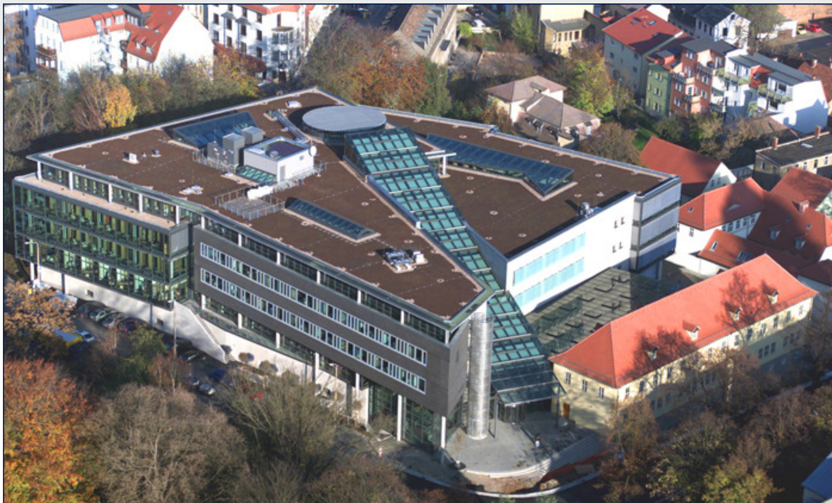
ThULB Jena: Main library building / branch library for Humanities
