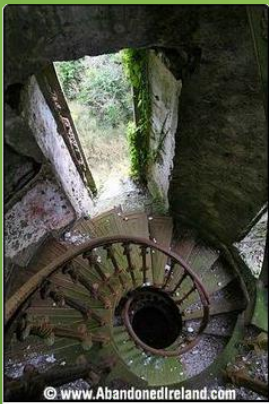
Abandoned ~ Foaty Tower, Co. Cork., Ireland
